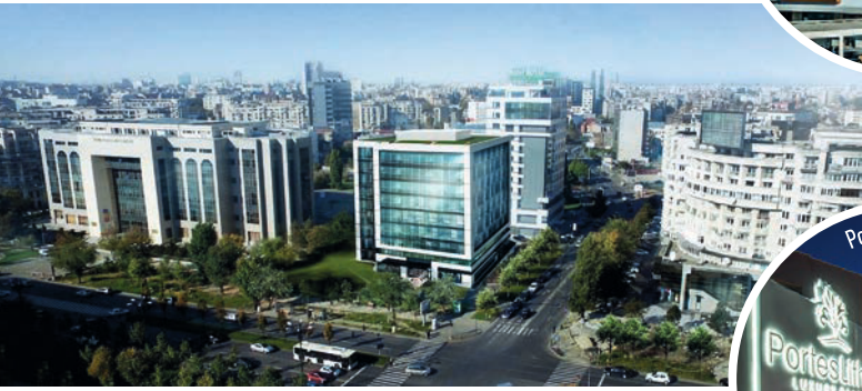
Day Tower - Office Building - Bucharest
